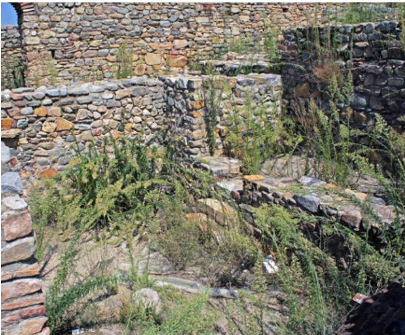
fig. 2. The Large thermae in Bargala, the open space where the relief was found, present situation
